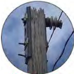
Pole Life systems WOOD POLE PRESERVATION
