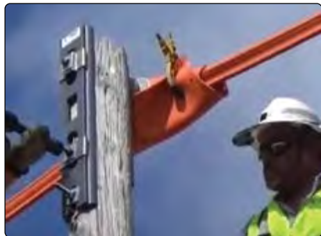
Pole Top Reinforcement - Vertical
