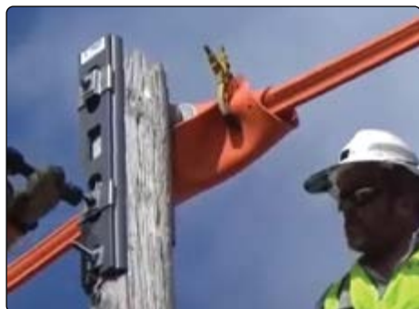
Pole Top Reinforcement - Vertical
