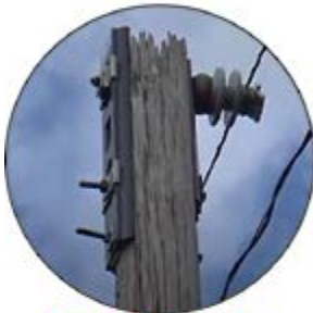
Pole Life systems WOOD POLE PRESERVATION
