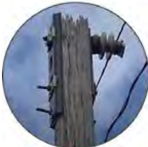
Pole Life systems WOOD POLE PRESERVATION
