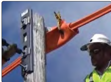
Pole Top Reinforcement - Vertical
