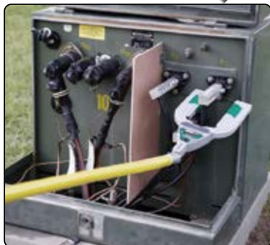
8-024PLUS Wide Jaw shown on Pad-mounted Transformer
