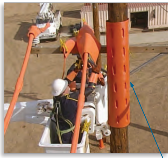
Strong memory improves grip when applied to the utility pole. The pole guard has high impact properties suitable for cold weather service.
