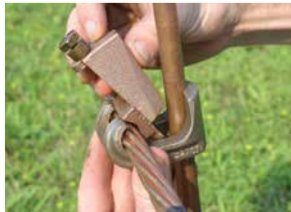
4) Insert wedge assembly while holding conductors in place.
