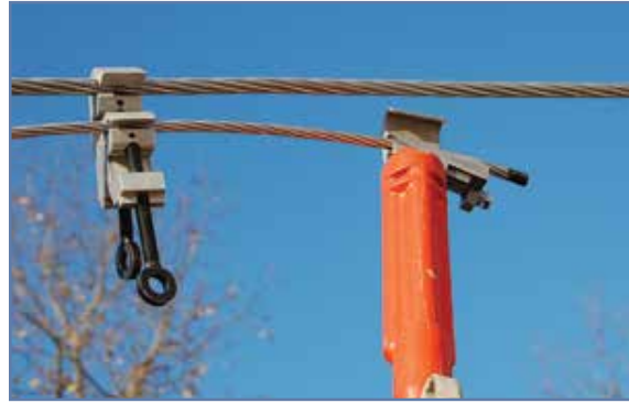
2) Place Tap Connector on conductors. Use Piggy-Back Clamp to hold conductors in place. Note: See page 22 for Piggy-Back Clamp ordering info.
