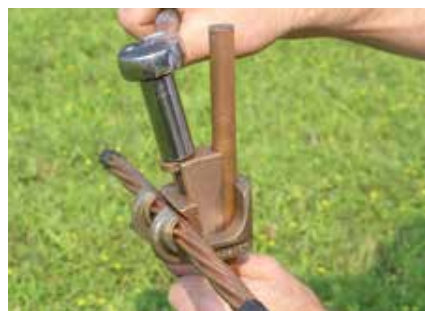
6) Use a 9/16" socket to drive the screw in.
