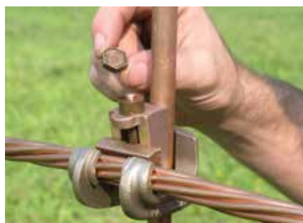
7) When shear head breaks off installation is complete. Any socket, speed, or impact wrench can be used.
