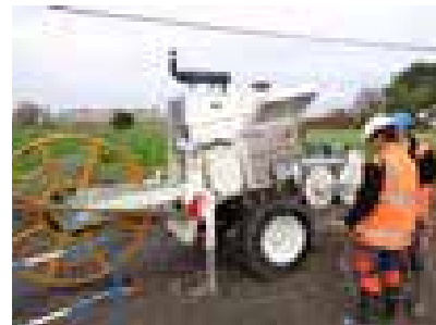
The "Dual Machine Concept" for both aerial and underground stringing operation
