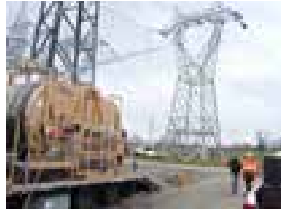
Twin puller tensioner with Ø 2 meter bull-wheels with interchangeable steel sectors and redundant hydraulic circuits
