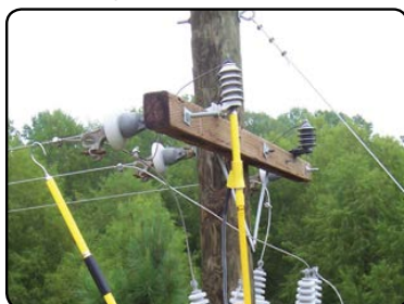
Lightning Arrester Testing
