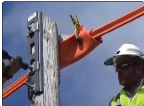
Pole Top Reinforcement - Vertical
