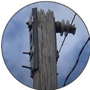
Pole Life systems WOOD POLE PRESERVATION
