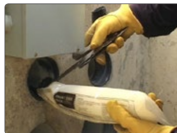
Polywater® Front End Packs lubricate ahead of the cable during the pull
