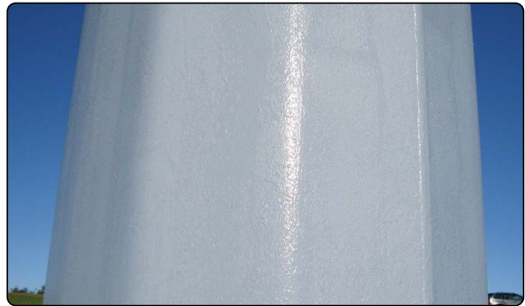
This 50-year-old rusty carbon steel pole was protected with an Induron coating system consisting of a SP-2 Hand Tool Cleaning, one coat of E-Bond 100 Penetrating Sealer, and 1 brush applied coat of Induraguard 9200.
