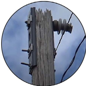
Pole Life systems WOOD POLE PRESERVATION
