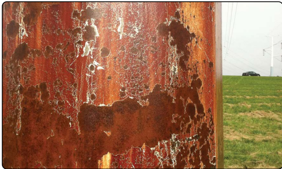
This 50-year-old rusty carbon steel pole was protected with an Induron coating system consisting of a SP-2 Hand Tool Cleaning, one coat of E-Bond 100 Penetrating Sealer, and 1 brush applied coat of Induraguard 9200.
