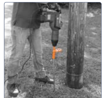
Then complete the driving by hammering from the top
