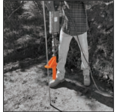
No ladder needed to drive rod.
