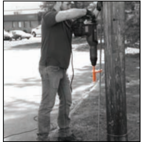
Safely drive rods from ground.
