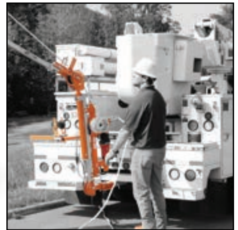
Pull overhead lines.
