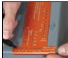
Step 1: Mark the first conduit.
