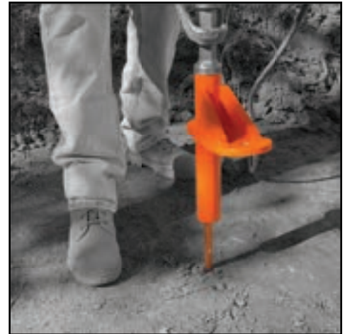
End receiver drives top of rod below grade.
