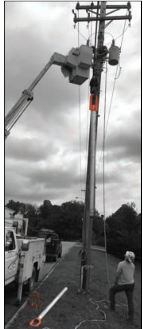
Conduit stays level for connection.
