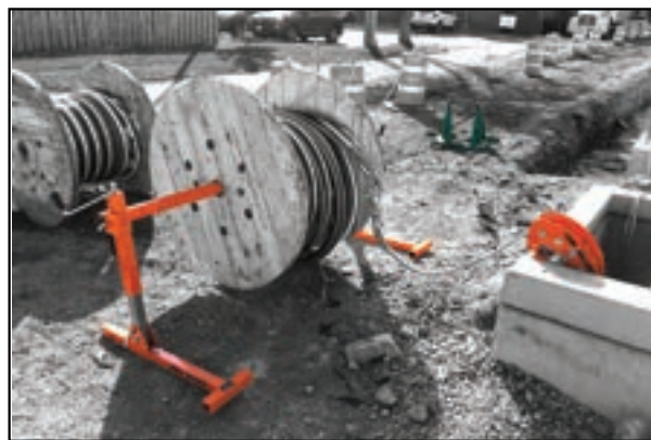
Separate sides can be used safely on uneven ground
