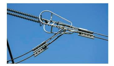
easily installed solution for restoring the electrical and mechanical integrity of connectors without the need for costly re-stringing or remediation works. With over 1000 units installed in Australia, ClampStar<sup>®</sup> is well on its way to helping Australian Transmission Authorities extend the life of their networks.
